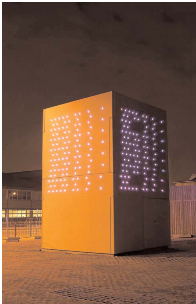
The new Pump House at Movers Lane
