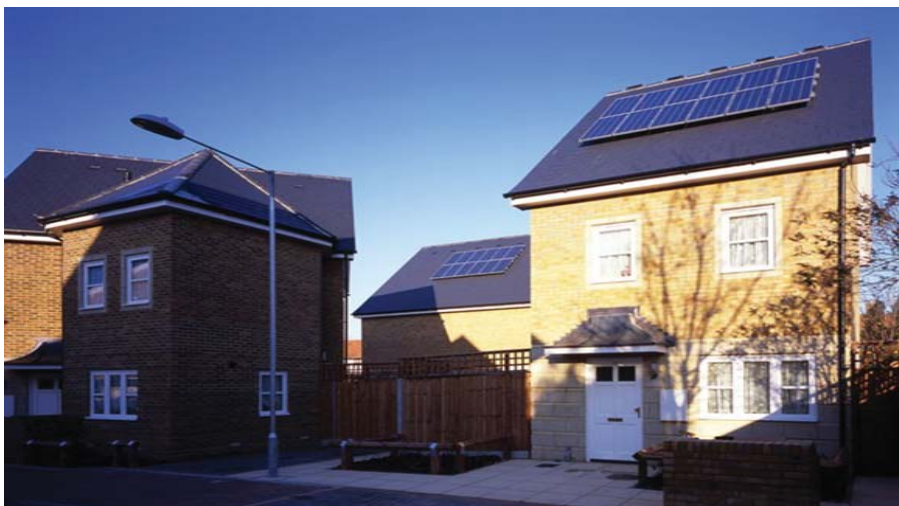
Charlecote Road development
